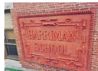
Terra Cotta Panel – 2 nd Flr
