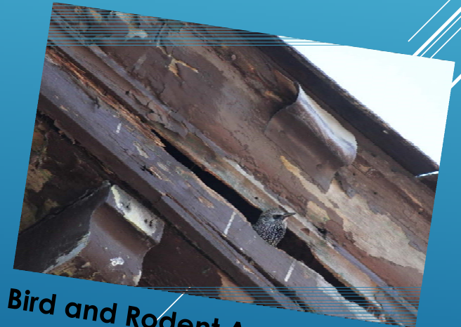
Cornice Structure Failing
