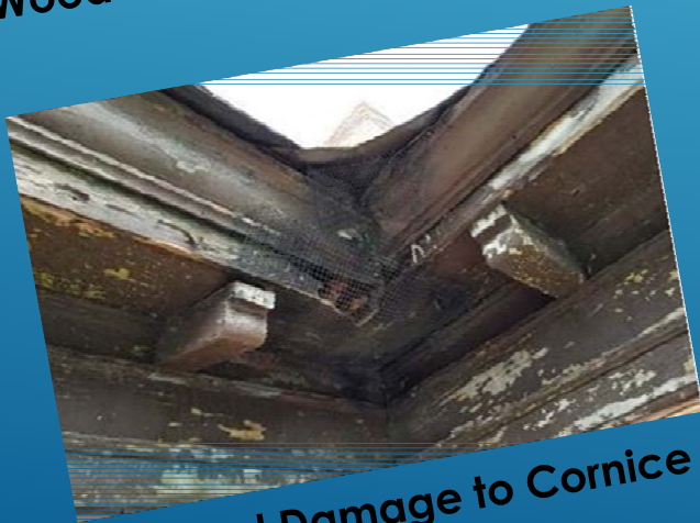
Wood Trim and Masonry Deterioration
