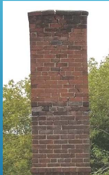
Cracked Chimney Removed
