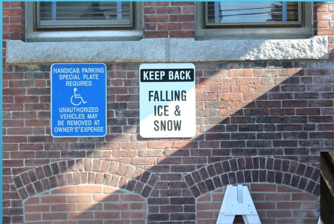
Falling Ice Snow Bricks & Slate
