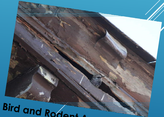
Cornice Structure Failing
