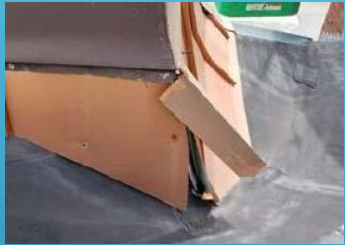
Damaged Flashing
