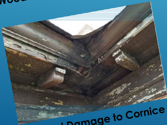
Wood Trim and Masonry Deterioration
